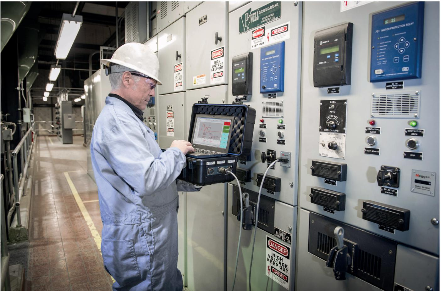
A technician using an EXP4000 analyzer connected to an EP1000 port at an MCC.
